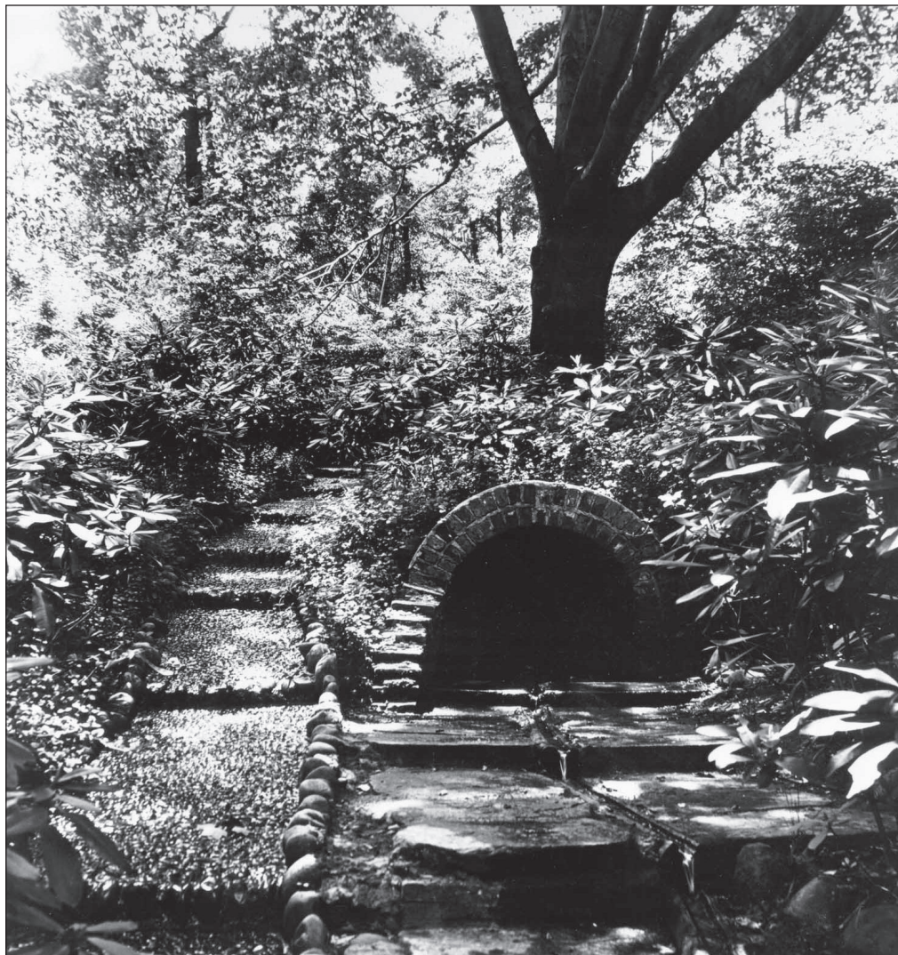
Figure 1.18 The pebble stream channel diverted storm water from the work yard down to the stream, while a natural spring emerged from the Spring Grotto and ran down the cedar rills to a cistern, c. 1935 (DOSLA Photo Archive, #13.21).
