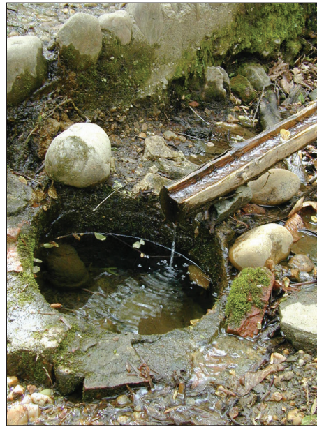
Figure 3.39 (left) Cedar rill detail directing spring water into circular well (NCR 2000).
