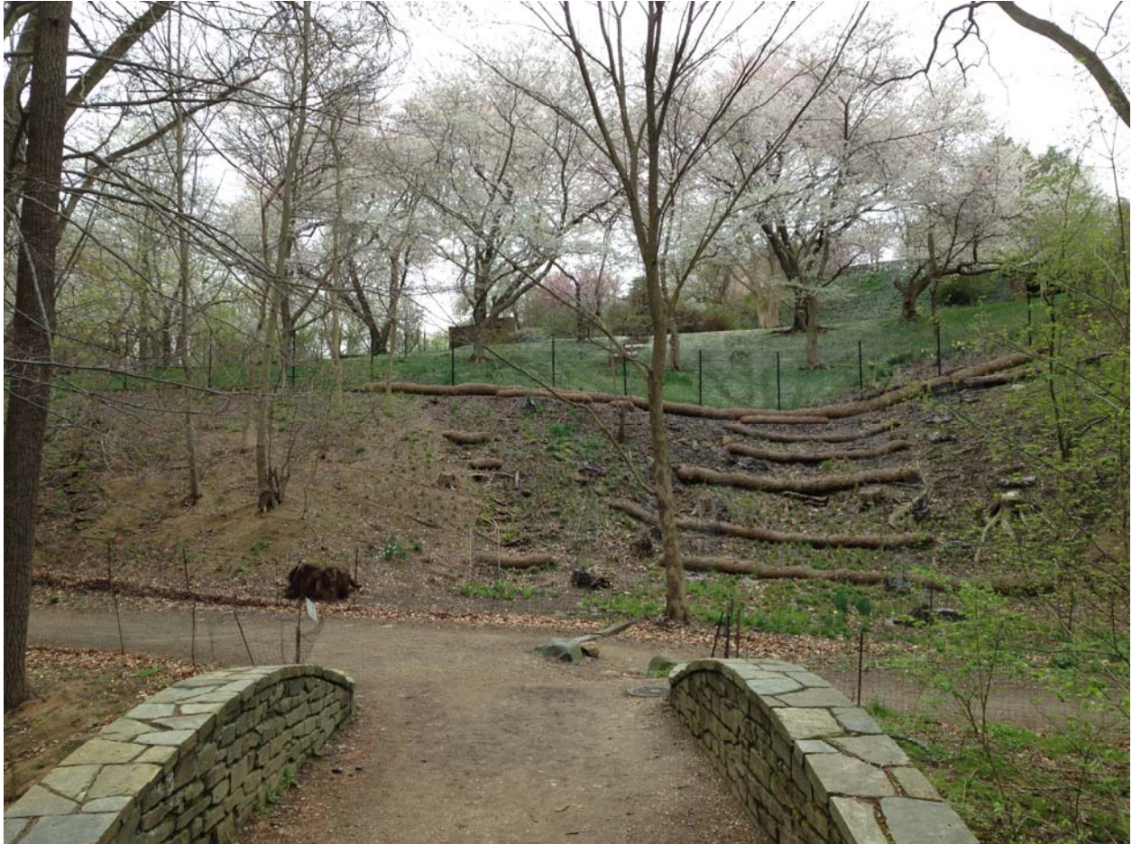
Figure 3 Compost logs and plant stabilization of Bridge Hollow, April 2015 (NCR CLP)
