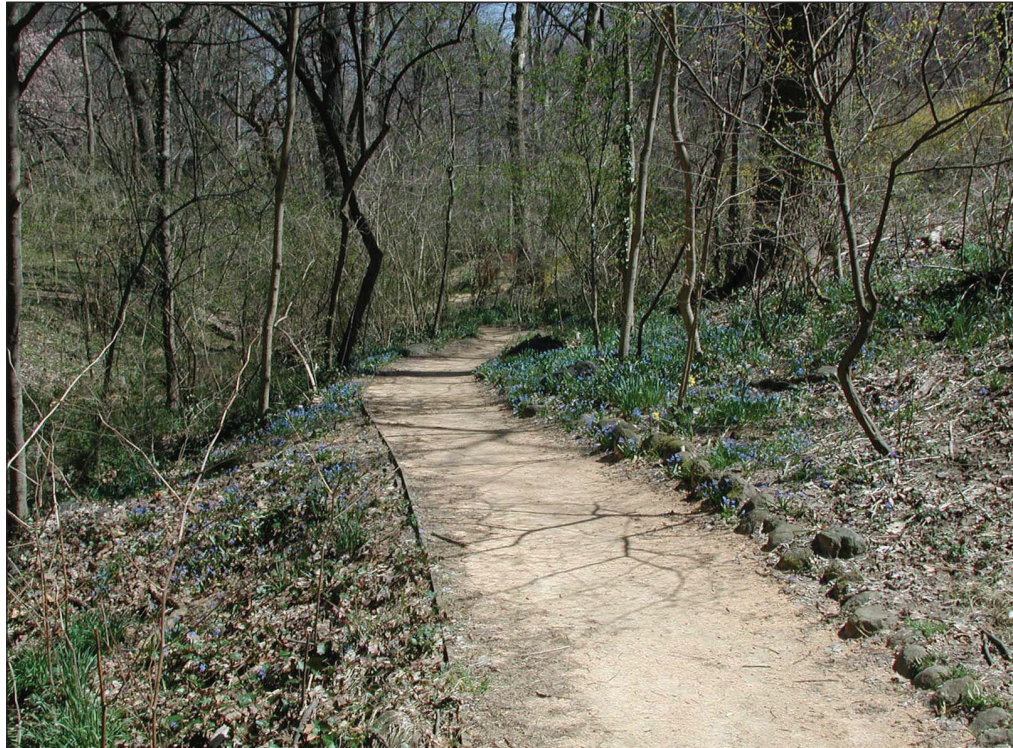
Figure 3.21 Intact portion of the south stream path between the stone bridge and Gray Arbor Memorial. The distinctive design features include the round edge stones on the uphill side, marker stones at trail intersections and a five foot wide stable surface (NCR 2005).
