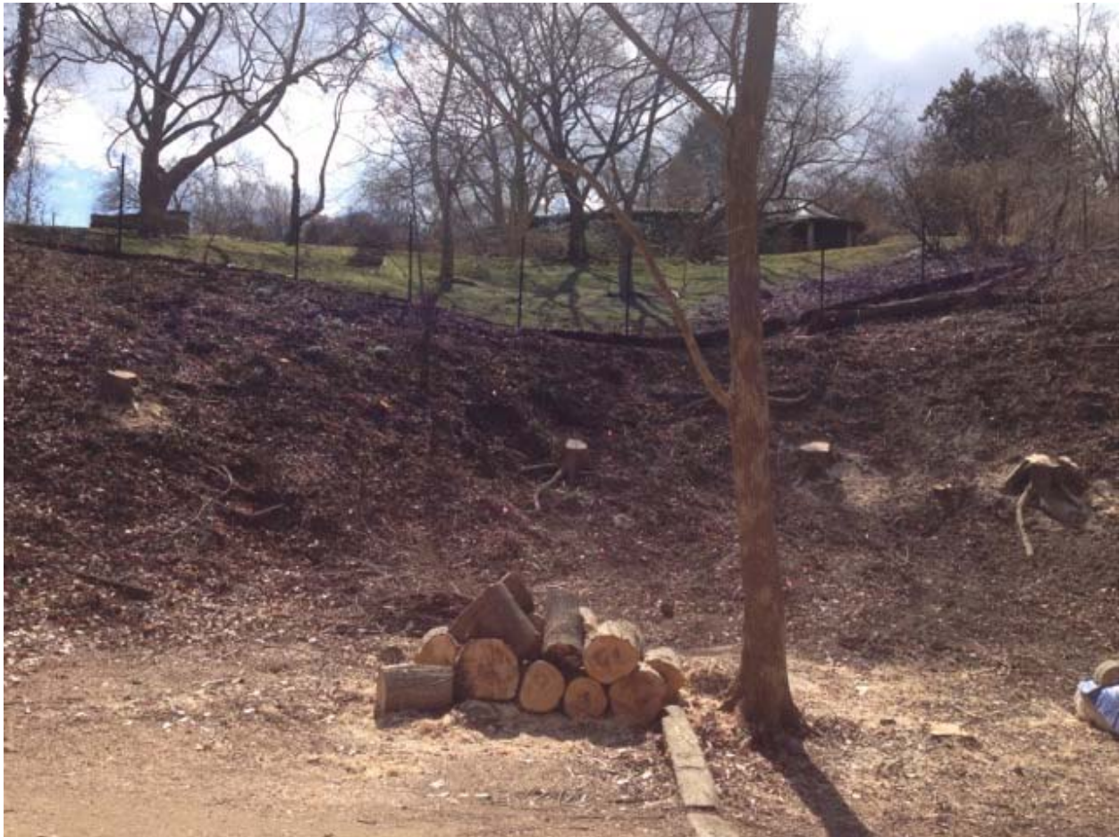
Figure 1 Bridge Hollow after removal of invasive vegetation and before installation of coir logs, March 2014 (DOPC)
