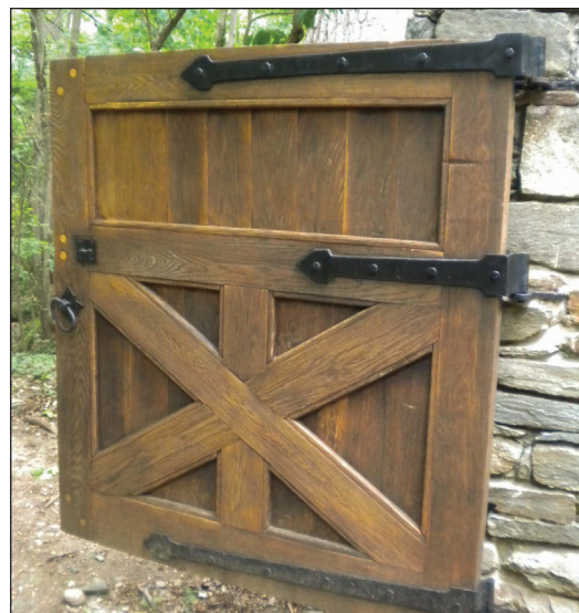
Figure 1.8 Replacement wooden gate used original strap hinges and lock (NCR 2012).
