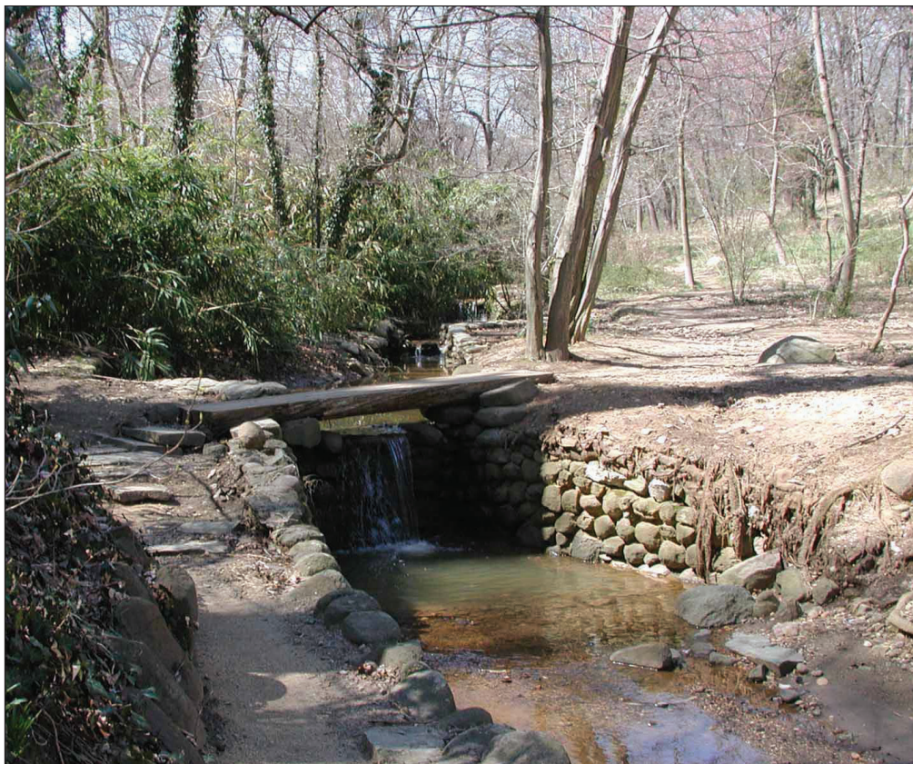
Figure 1.17 Rustic oak logs were salvaged from downed trees in Rock Creek Park to reestablish the log bridge crossing at Clapper Bridge Falls (NCR 2005).
