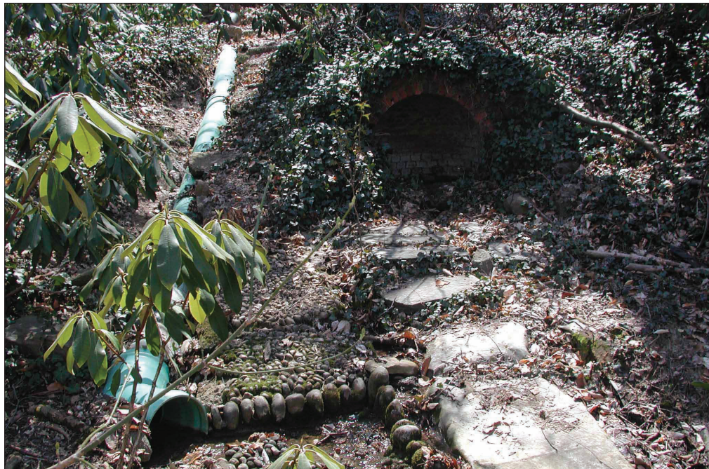
Figure 1.19 Temporary pipe routes the storm water further down the slope to a lower panel. The Spring Grotto no longer has an active spring running, so the cedar rills were removed (NCR 2005).
