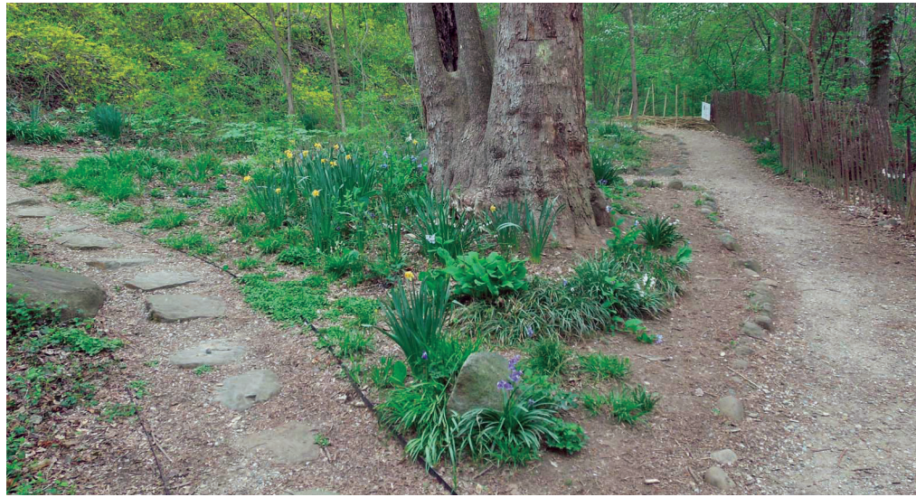
Figure 3.46 Edging and marker stones have lost their definition at critical locations (NCR 2013).
